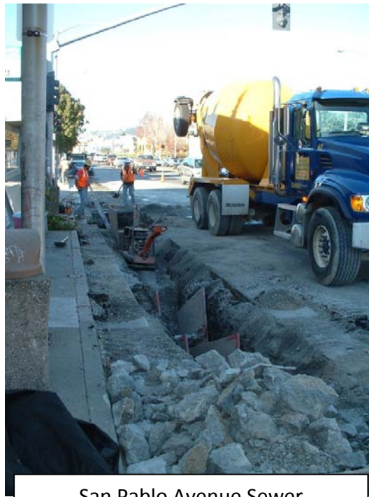
San Pablo Avenue Sewer
