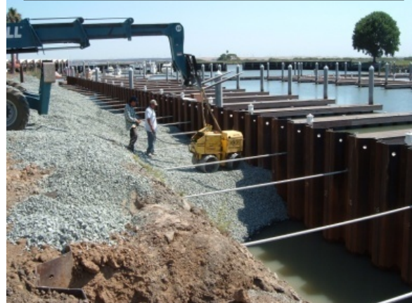
Pittsburg Marina Bulkhead
